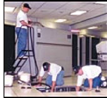
Typical sub-floor cleaning
